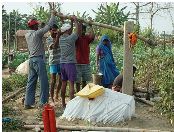
Figure 7: Farmers, from Mainhiya Village Development Committee, installing a treadle pump for irrigation. Photo: Practical Action Nepal / Matrika Sharma.
